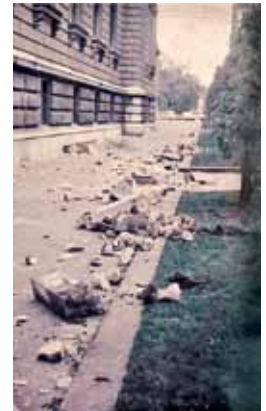
Building damage in Vienna 1972
