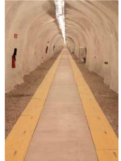
Main tunnel of the geomagnetic observatory.
